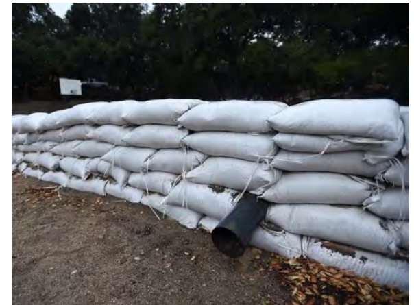
Kagel Canyon Precipitation Preparedness and Mudslide Prevention - Jan 2018 Source: Flickr, CEO Countywide Communications
